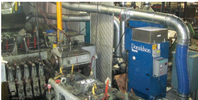
WSO on Smoke - Cold Forming 1,200 cfm (2,038 m³/h)
