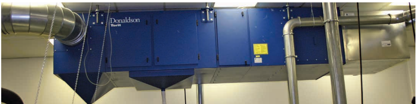
MODULAR MEDIAFILTER™ on Grinding 2,000 cfm ( 3,397 m³/h)
