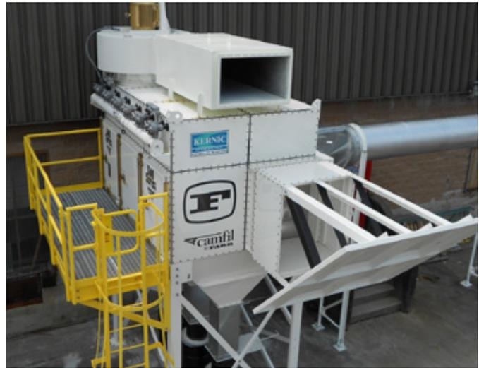
*This dust collector is equipped with an explosion vent with vertical upblast deflector plate. Other safety features include a sprinkler system and filters with special carbon-impregnated media for static dissipation.*
